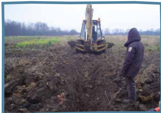
Breaking drain tile for wetland restoration — MMSD
