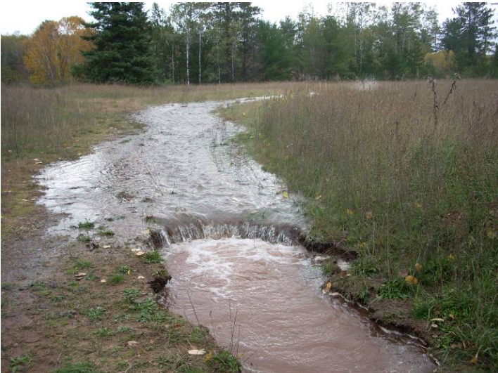
Eau Claire River, DO-S22, Overland Pump Around Scouring Report 1b-ST-015 – 10/11/07
