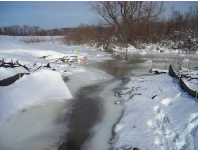
MP 317.3. Silt fence does not extend across entire disturbed ROW Report 4-DD-102 - 2/7/08
